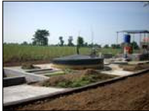
Biogas based power plant
