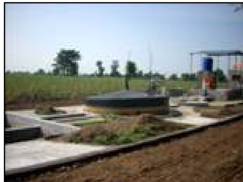
Biogas based power plant
